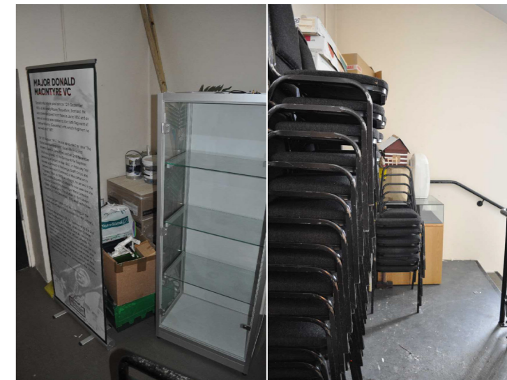
Existing - Items stored in and on escape stair
