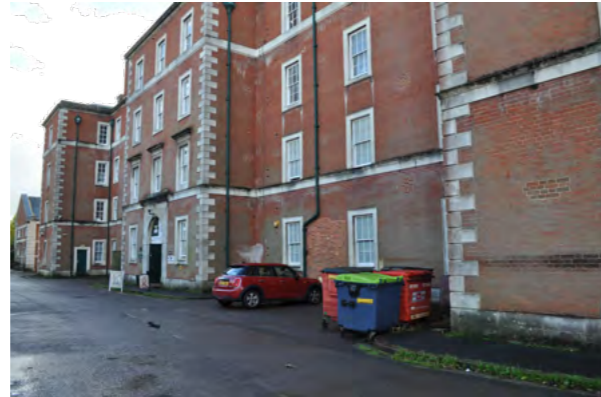
4 - Rear entrance area used to store bins and is poorly maintained.
